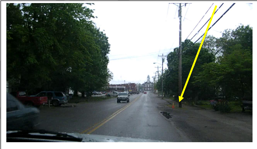
Photos 3 & 4: Access, Sidewalk & Drainage needs
